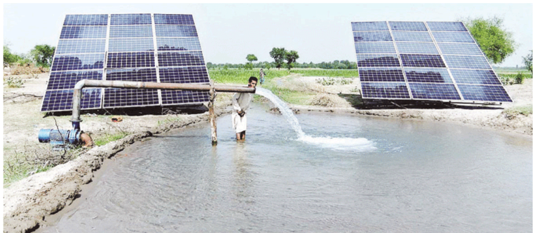
CHINIOT: Solar panels installed for running a tube well.--APP
