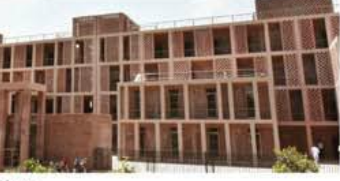
Extension block of Razia Hassan School of Architecture
