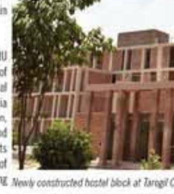
Newly constructed hostel block at Tarqil Campus
